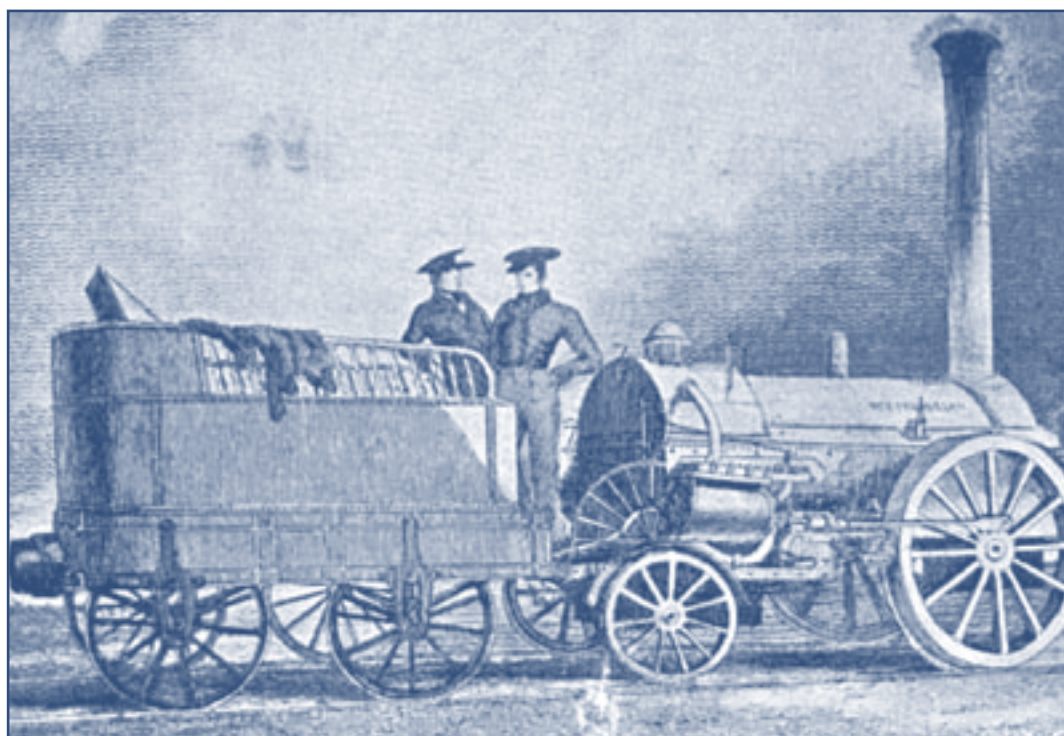
Above - Robert Stephenson’s “Northumbrian”, Liverpool and Manchester Railway, circa 1830. An example of outside cylinder type.
