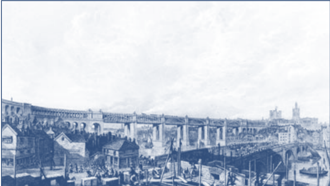
The High Level Bridge
